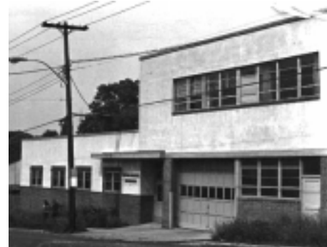
First site of Yonkers Center on McLean Avenue.
